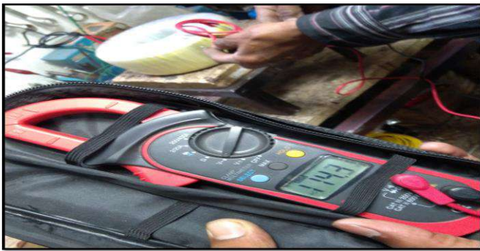
Fig. 2.3: Toroidal Transformer input & output
